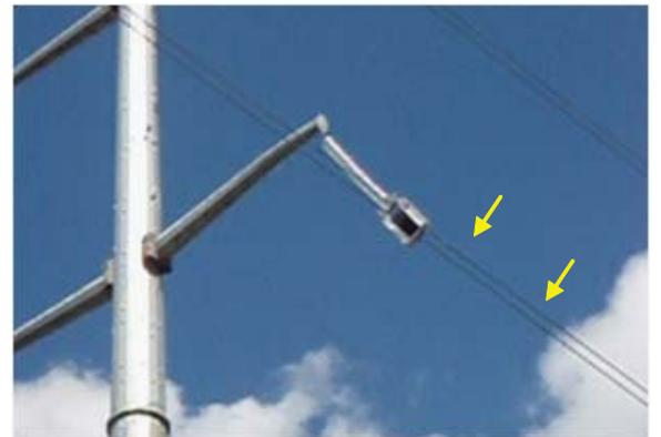
Two IMPLO splices easily pass through the stringing block on their way to final placement in the line.
