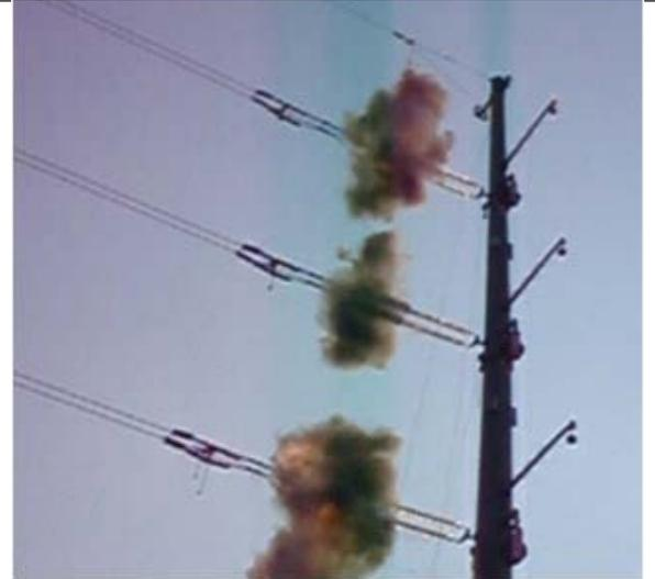
Six IMPLO deadends are safely installed all at once, increasing productivity. Glass insulators are not affected by the proper installation techniques.
