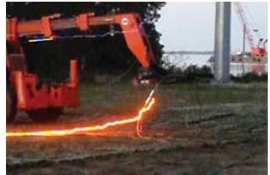
An IMPLO ACSS splice is ready to go. The non-electric shock tube glows brightly for an instant just before the sleeve installs. The installation process is very safe and environmentally friendly.
