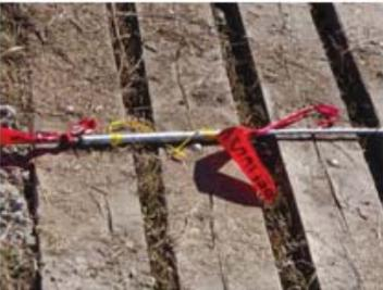
An IMPLO 7/16" static-wire splice is brightly tagged so that it may be easily located for inspection when pulled to its final location.
